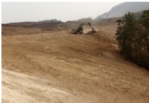
Hinsom Valley – topsoil spreading
