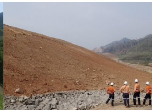
Phabing C backfill – topsoil cover
