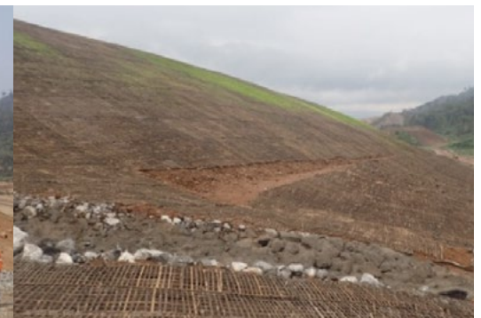
Phabing C backfill – first stage rehabilitation
