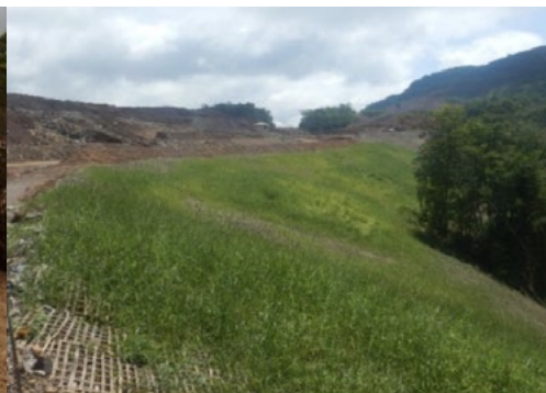
Hinsom Valley – second stage rehabilitation
